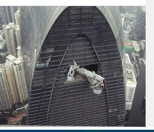
Acknowledged as the world's most energy-efficient 'green' building, the gently curved Pearl RiverTower is constantly in the public spotlight and media. Architects Skidmore, Owings & Merrill designed mechanical floors with funnel-like openings at approximately one-third and two-thirds of the way up, to house wind turbines that generate energy for the building.
